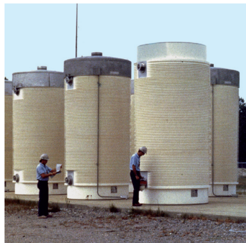
Figure 2-1. Dry Storage of Spent Fuel (Source: NRC 2013b)
